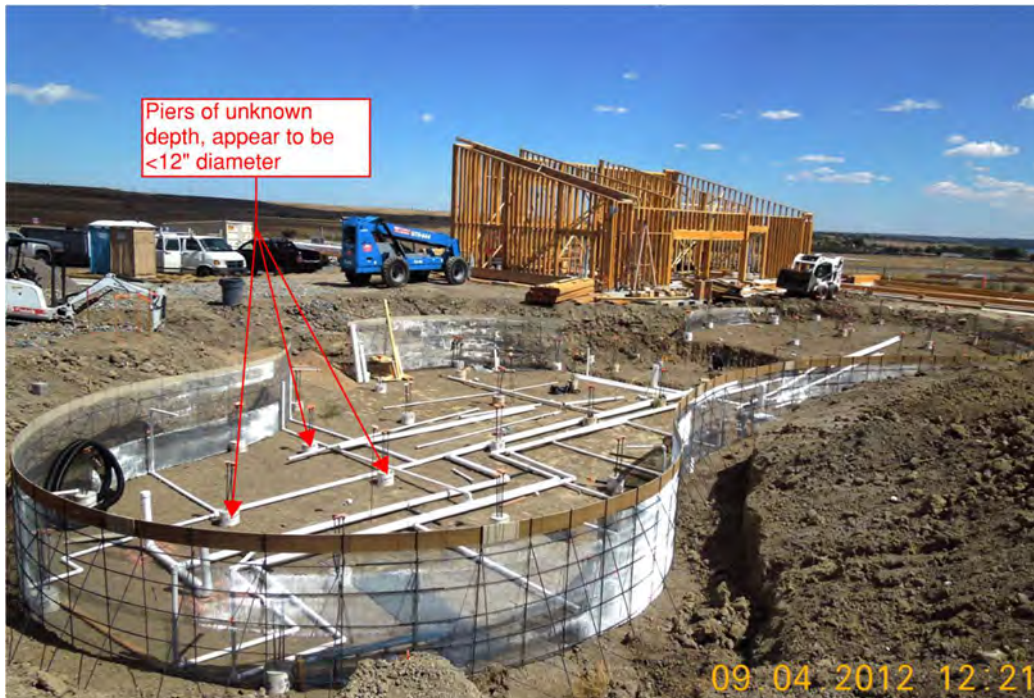
Figure 1 – Photo taken during construction of the Townview Community Center Facility
